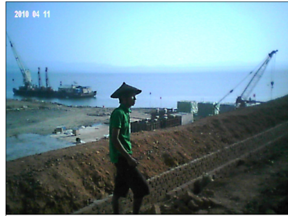
The deep-sea port construction site at Maday Island, Arakan State.
